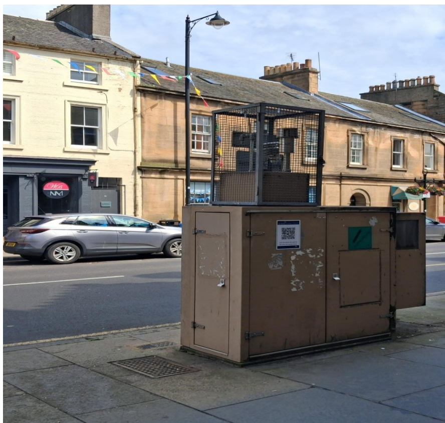
Linlithgow Automatic Continuous Monitoring Station – High Street Linlithgow
