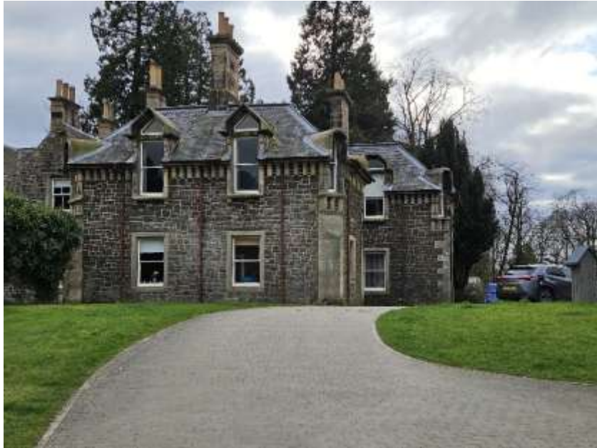
Figure 6.2: Gowan Bank House sitting prominently within the conservation area
