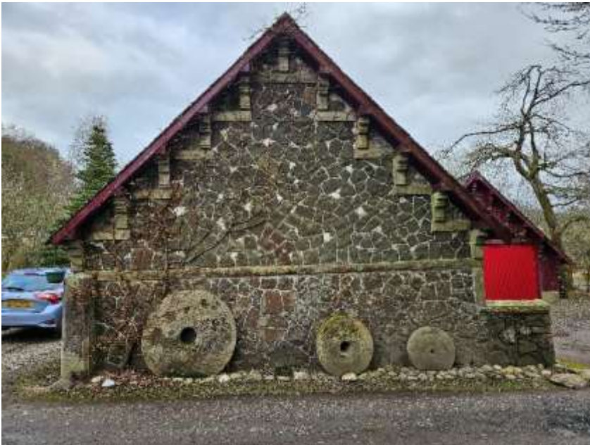
Figure 6.5: Gable end of building showing rubble masonry
