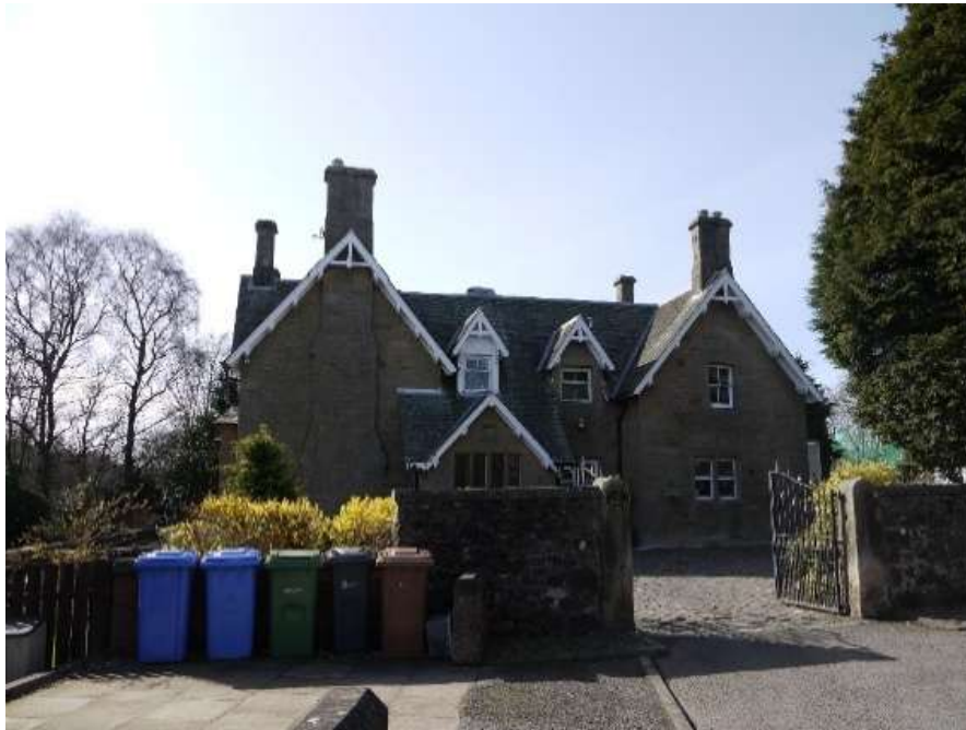
Figure 6.30: Villa in Forkneuk Road with picturesque roofline and details
