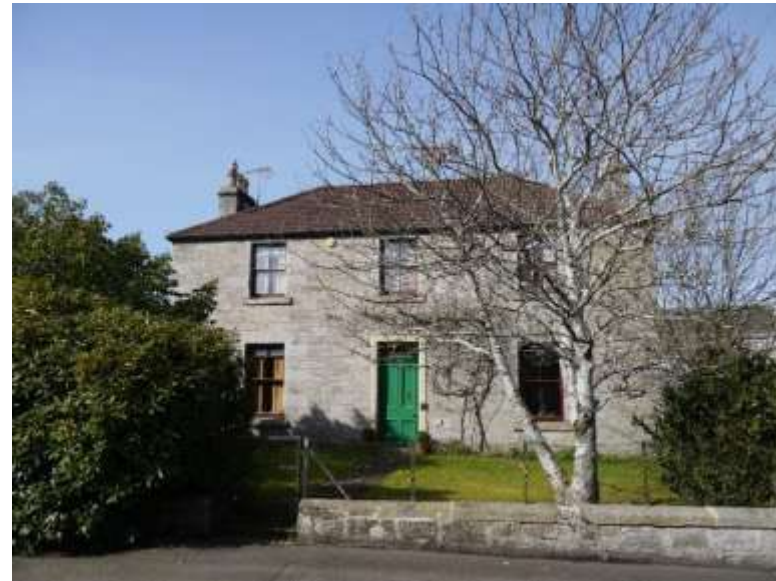
Figure 6.14: Stone boundary wall and front garden, Forkneuk Road
