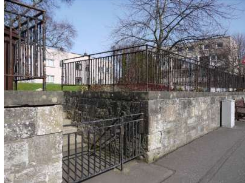
Figure 6.35: School Place, set within landscaped grounds
