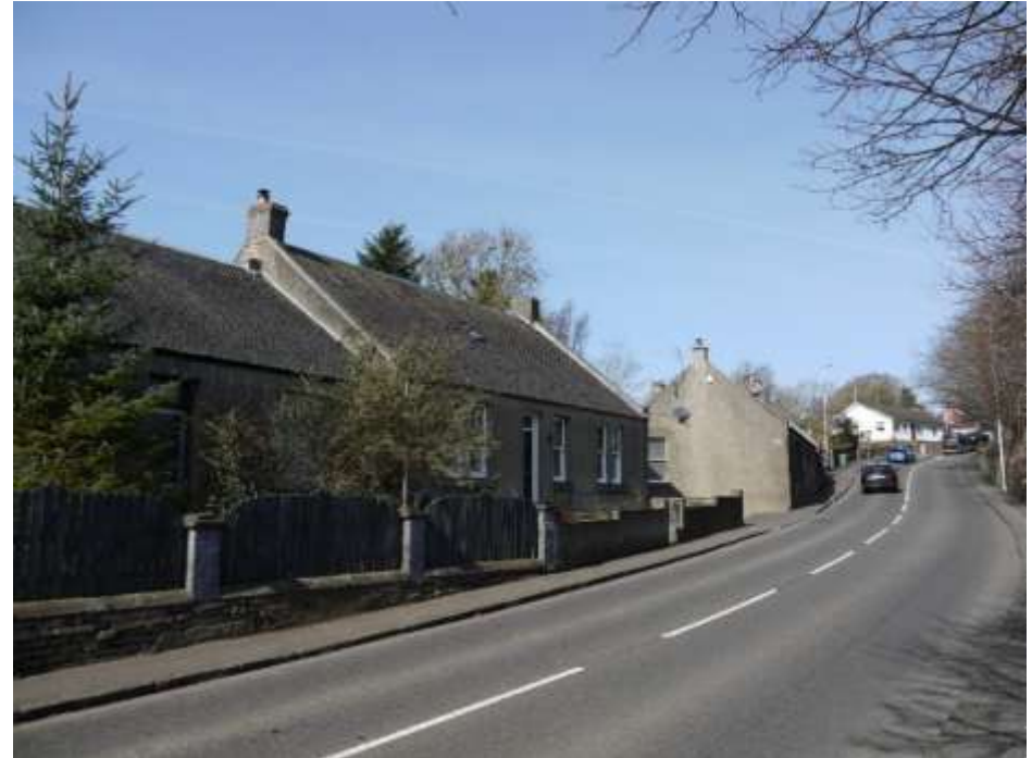
Figure 6.16: Winding Ecclesmachan Road rising towards Uphall Kirk
