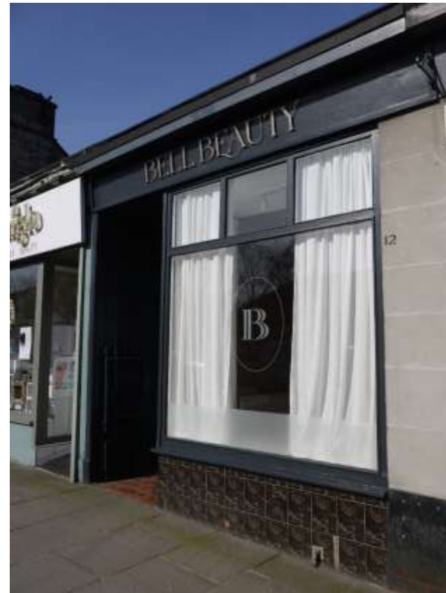
Figure 7.1: Good examples of shopfronts
