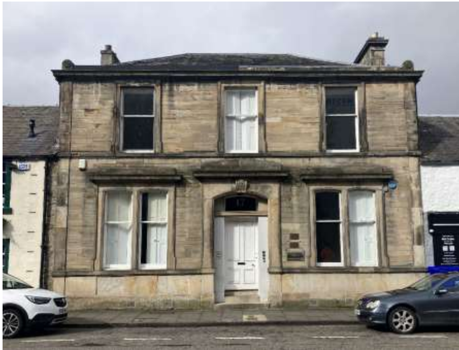
Figure 6.12: Plate glass sash and case windows, panelled timber door, shutters, finishes and architectural detailing, Bank Street
