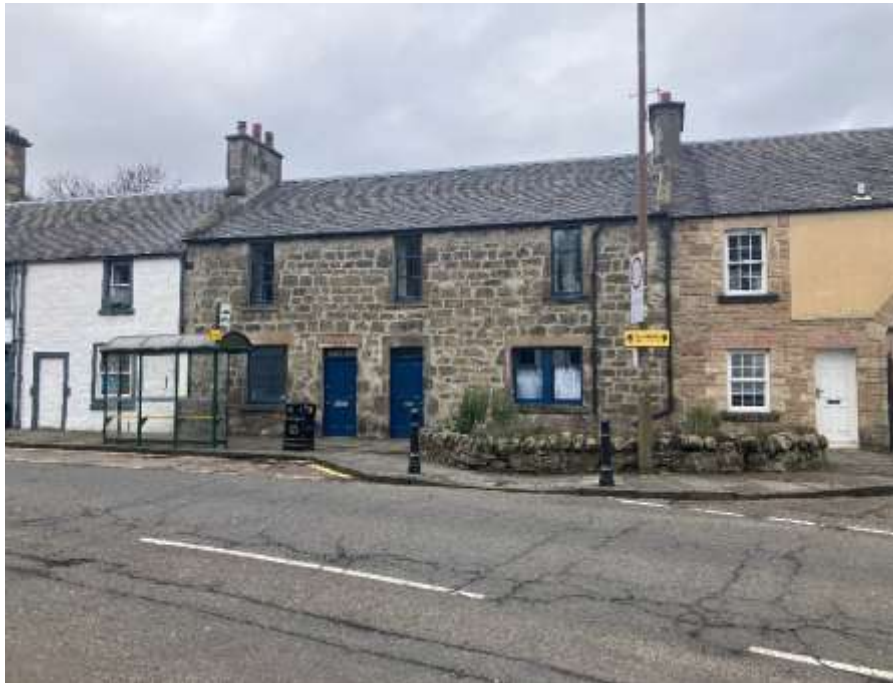
Figure 6.10: Group of two-storey houses, Bank Street
