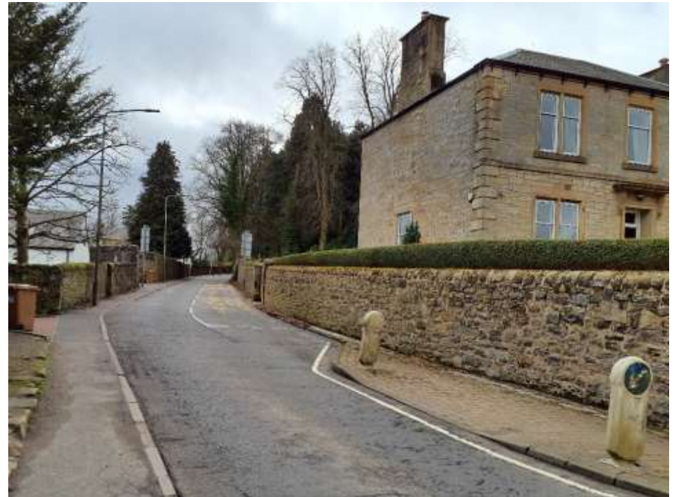
Figure 6.13: Rubble boundary walls define villa gardens and enclose the road, Pumpherston Road
