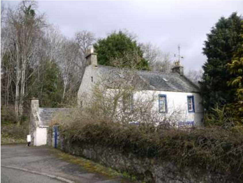
Figure 6.25: Harled villa with traditional outbuilding and boundary wall, Pumpherston Road
