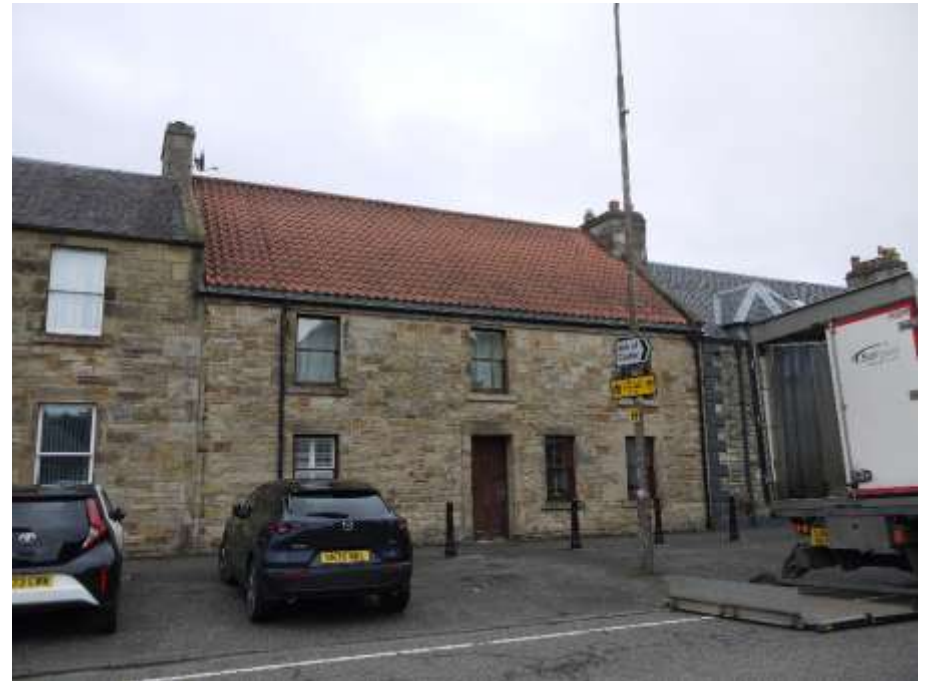
Figure 6.11: Two-storey traditional building with pantiled roof with easing course, Market Street
