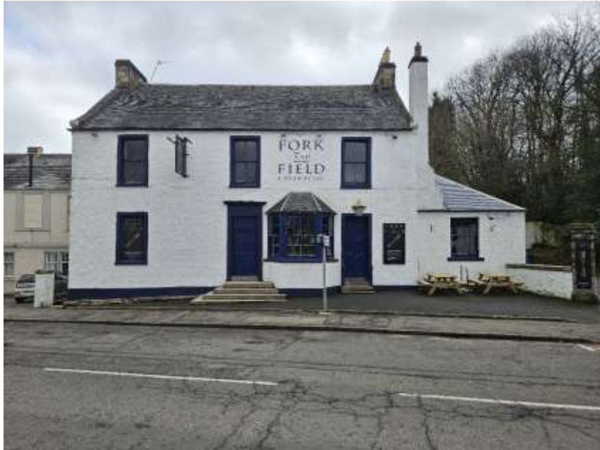
Figure 6.21: Fork and Field, the former Torphichen Arms, Bank Street
