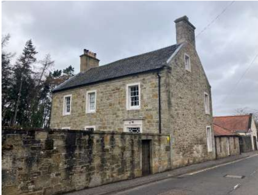
Figure 6.23: Two-storey villa with pantiled outbuildings and high rubble boundary walls enclosing garden, Main Street
