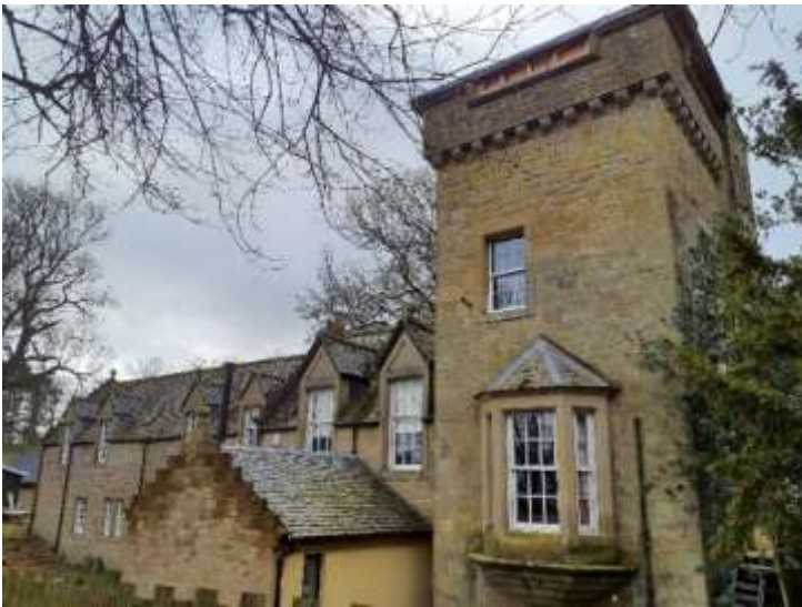
Figure 6.11: Two-story tower lodge with corbelled parapet, angle turret, and a single storey addition
