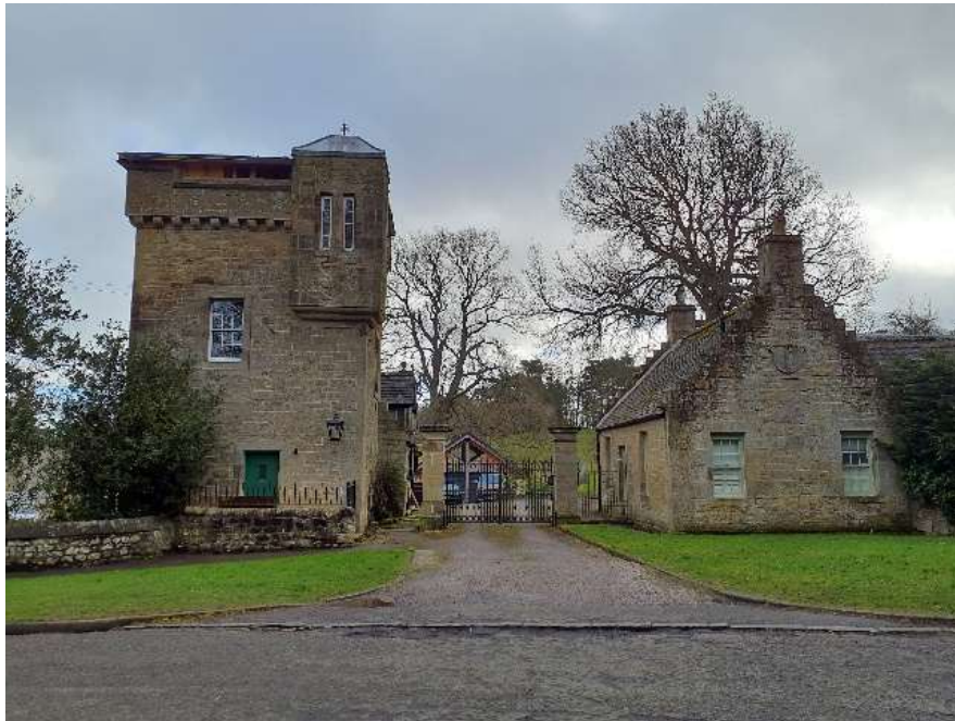
Figure 6.5: Lodges 19 and 21 Whitemoss Road (LB7348) stand prominently at Whitemoss Road
