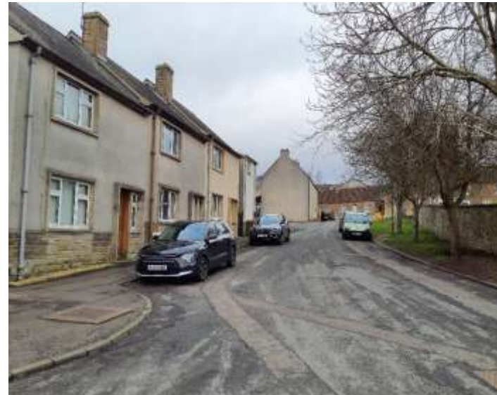
Figure 6.12: 20 th century houses at the south end of Smithy Brae
