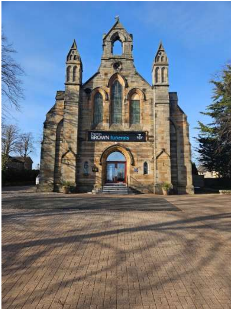
Figure 6.3: The stature of West Church, 18 West Main Street combined with its large plot allows it to form a prominent landmark
