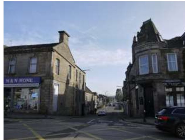
Figure 7.1: Well maintained road with development maintaining the historic linear nature of development
