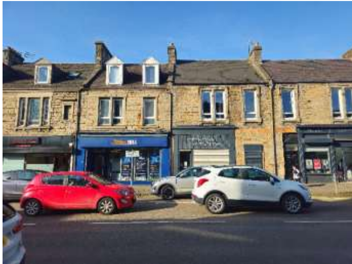
Figure 6.12: Row of properties with a consistent roofline and varied commercial premises below.
