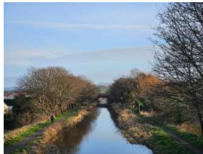
Figure 6.6: View along the Union Canal from the Main Street bridge towards Union Canal Bridge 25 (LB14231)
