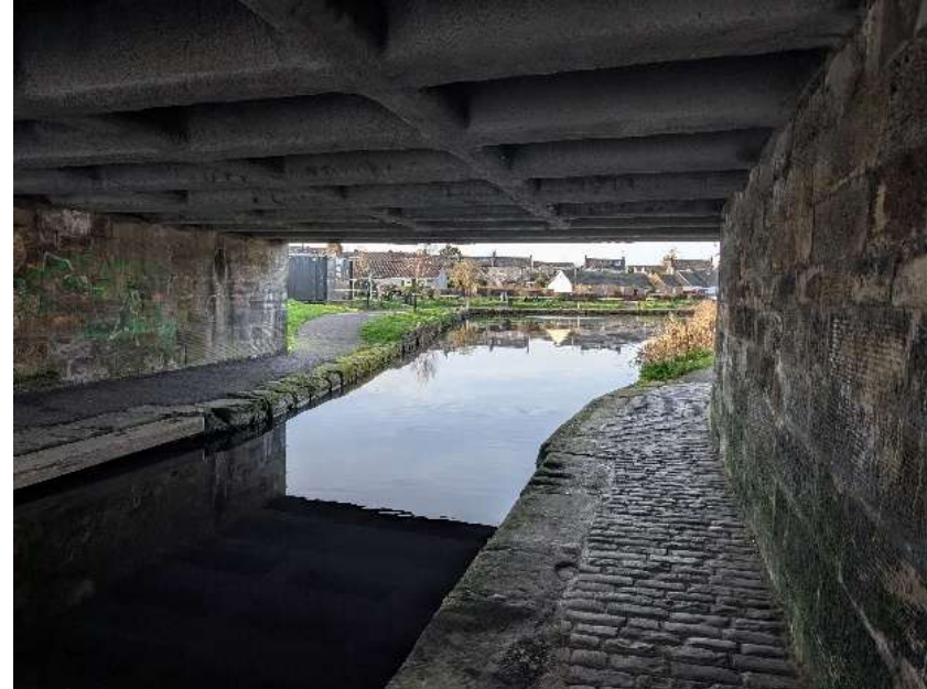
Figure 6.2: The Union Canal from under the bridge carrying the A899
