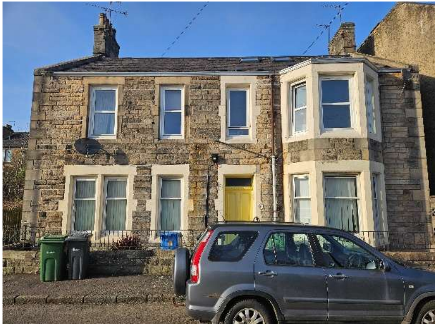
Figure 6.10: Building with painted margins
