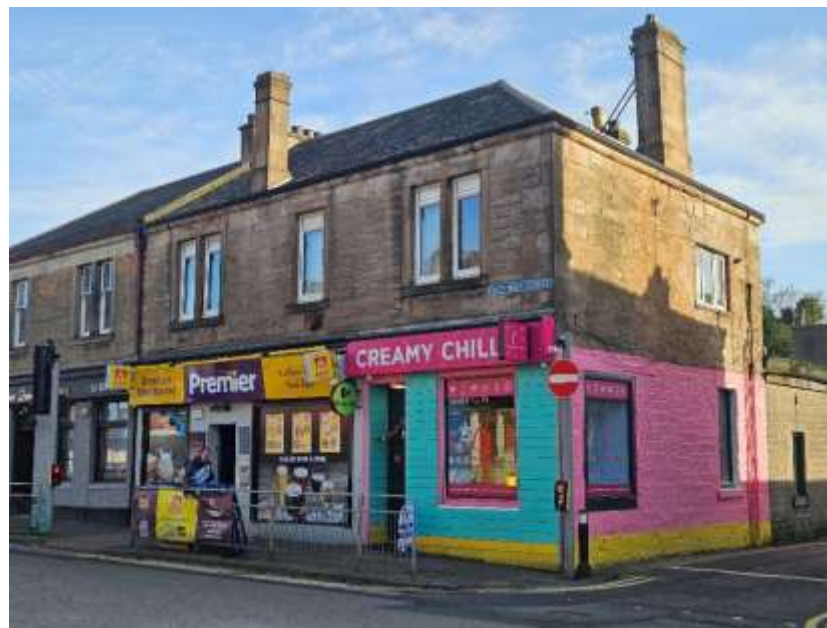
Figure 7.3: An example of an inappropriate shop front
