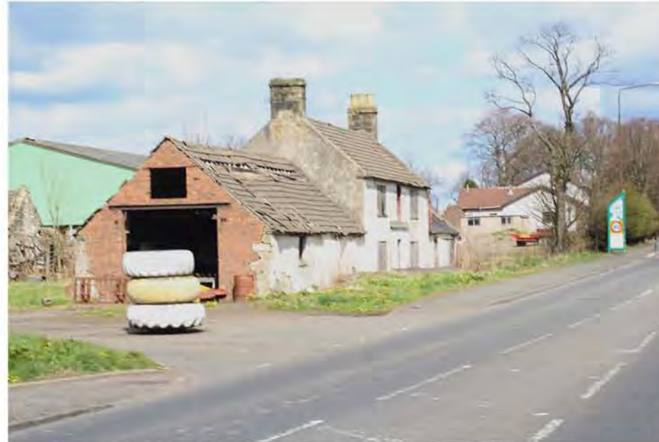
Derelict Farmstead on Redhouse Road
